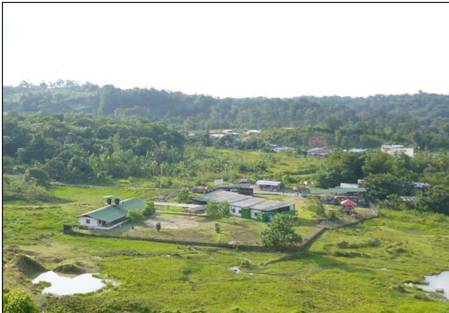
Figure 2: Novita Exploration and processing compound March 2015. Finished accommodation block and helicopter pad clearly visible on left side of compound (completed late 2013).
