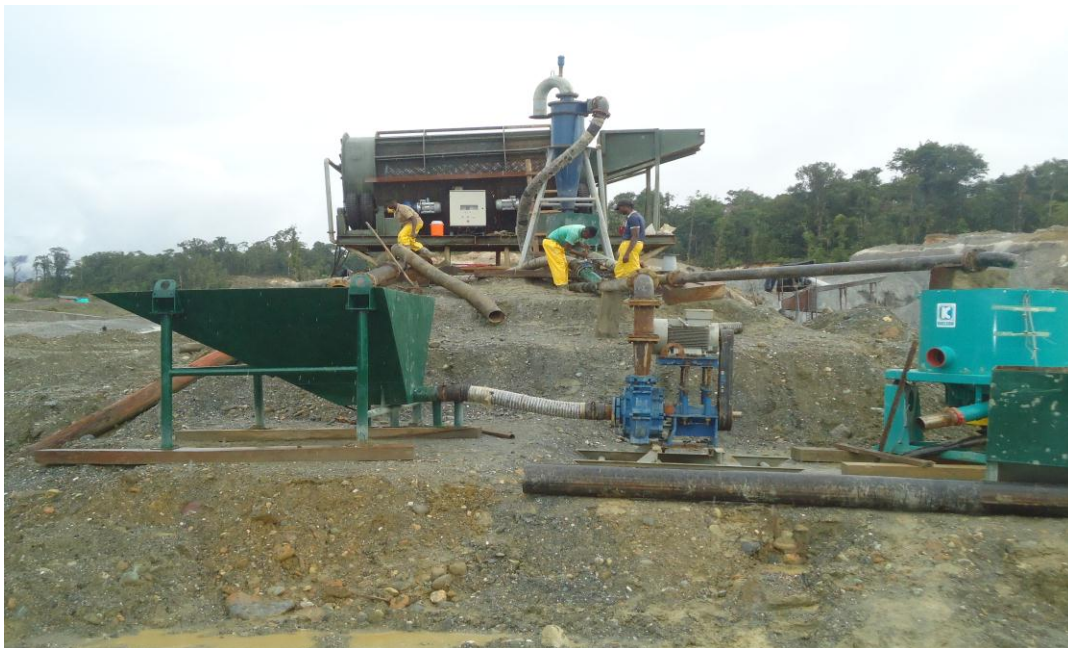
(Construction of Bulk Sampling Circuit)
