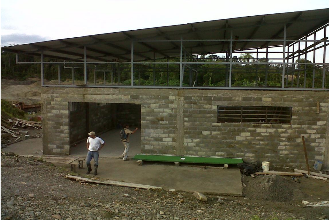
(Construction of Gold Room)
