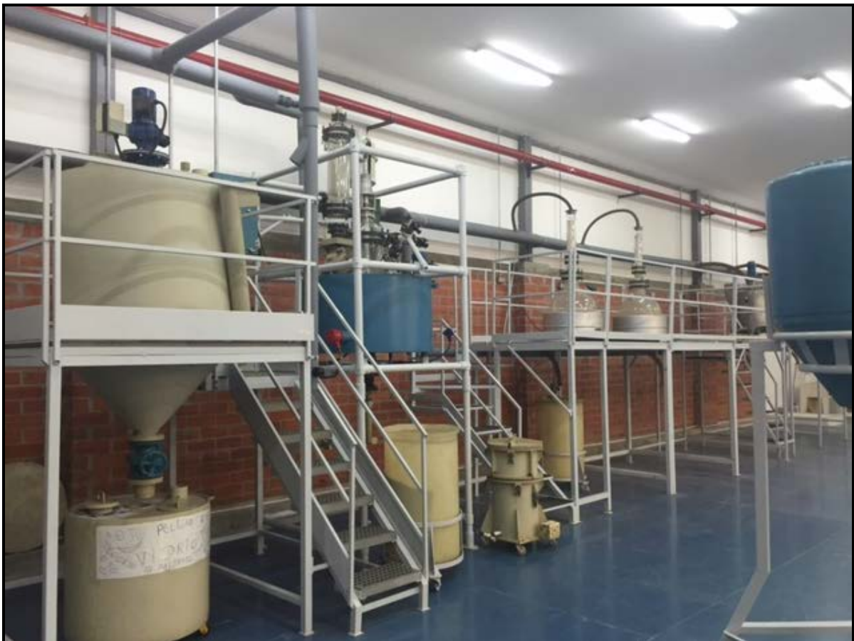
Fig 3: Section of refining circuit being installed at Cali facility
